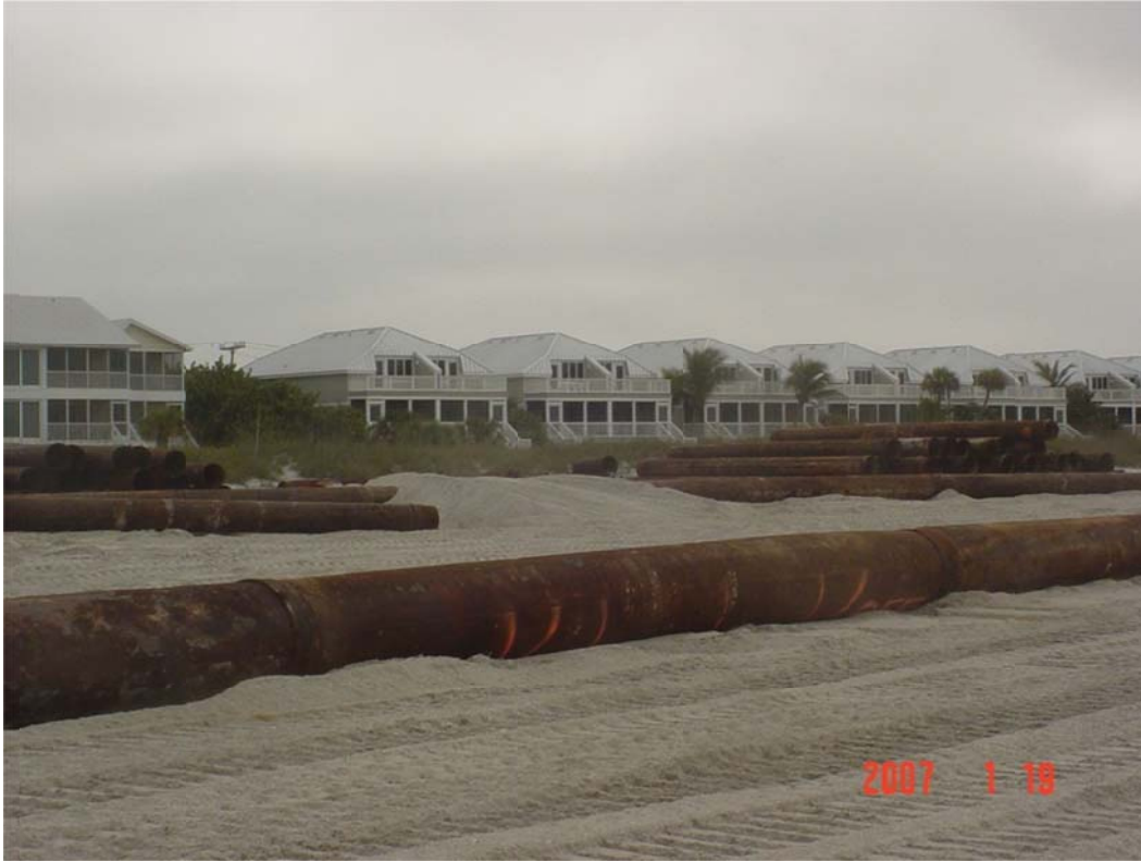
Typical View of Staging Area on the Beach
